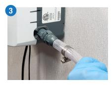
Connect 1/2" braided tubing (964800) to the water outlet and then run tubing to washing machine.
