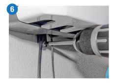
To secure the dispenser at the bottom, mark the hole location and secure with the remaining screw.
