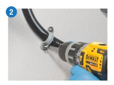
Install wall supports for the incoming water supply hose. This will prevent unnecessary force on the inlet fittings.
