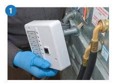
Connect the machine interface to the washing machine and install the controller.
