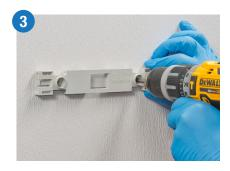
Attach the mounting bracket to the surface.
