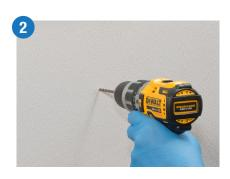
Drill holes in mounting surface. Use anchors where appropriate.
